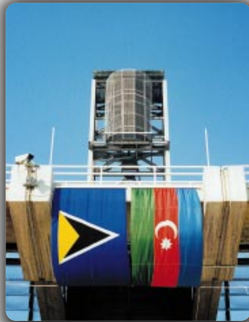
This small array consisting of just 25 KF900 modules fills the 85,000 seat Athens Olympic Stadium. Except in areas masked by overhung balconies, no additional loudspeakers were required.
